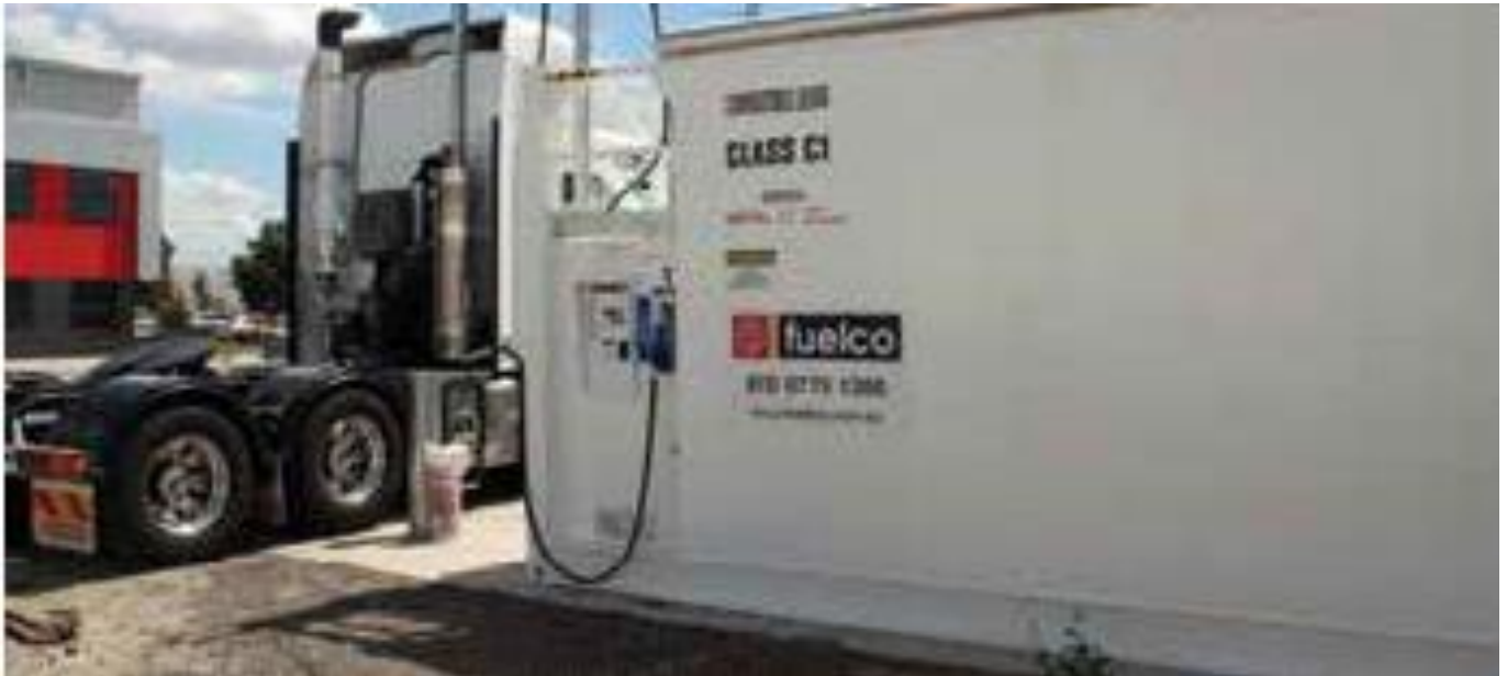
Figure 16.1. Self-bunded fuel storage tank with safe storage limit of 55,600L.
